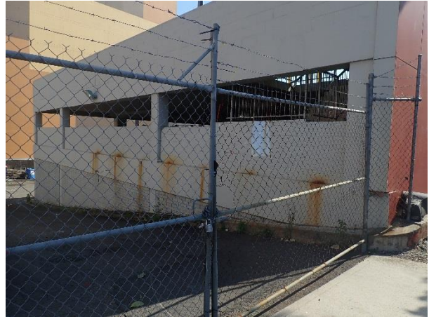
Plate 2. The multi-storey carpark on Terminus Street, cut into the slope of the hill.
