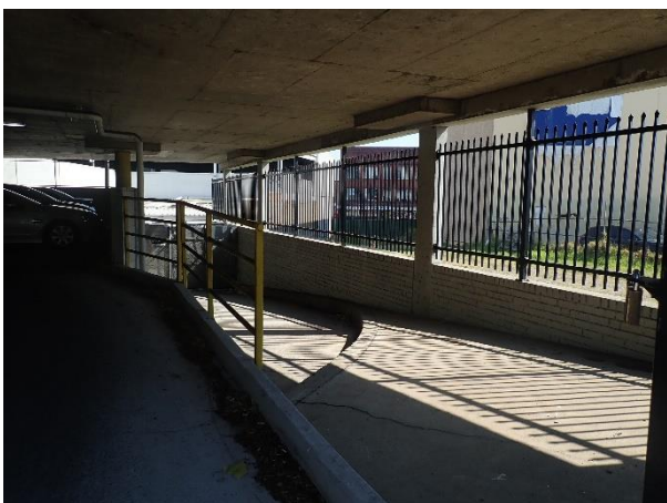
Plate 5. The interior of the carpark, further evidencing the highly truncated nature of the area.
